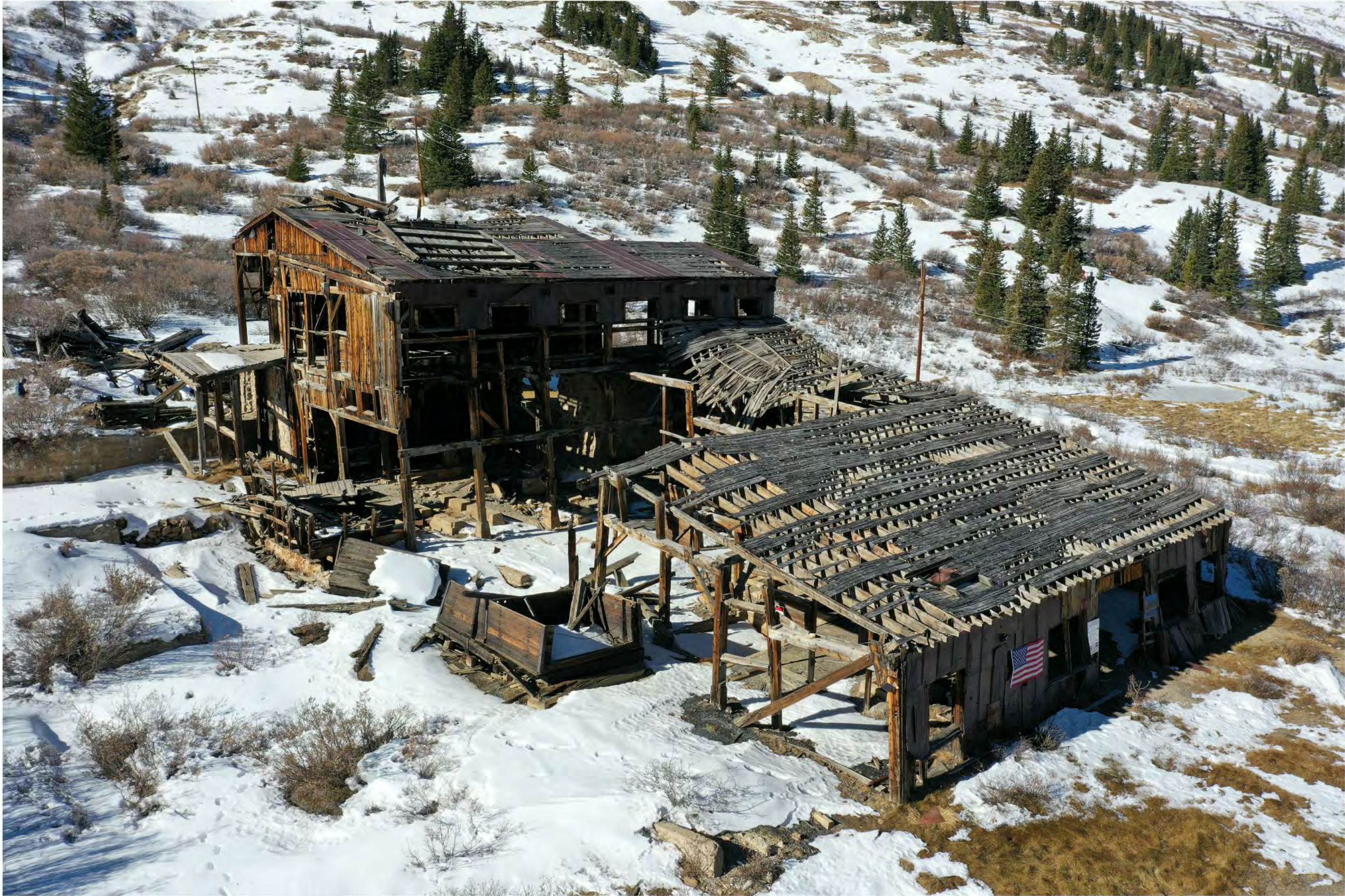
1 ROOF AERIAL S001 NO SCALE
